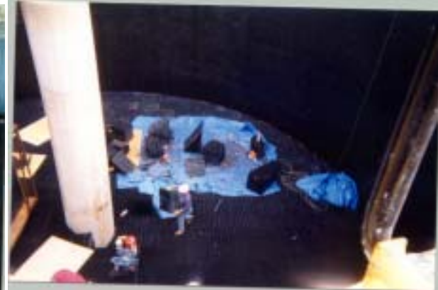
Tarped cutting area with plywood under the tarp
