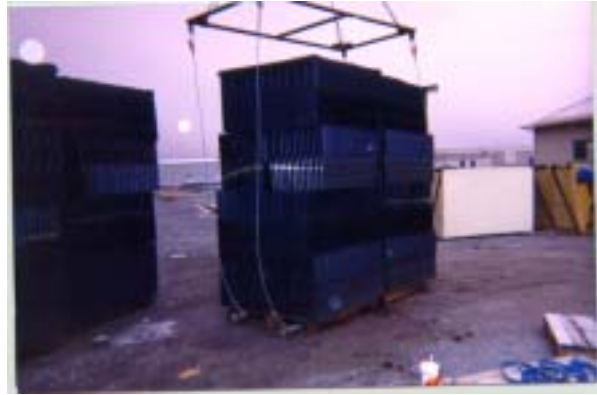
Pipes w/D-rings & quick-release cables
