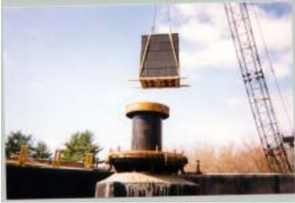
Rigging using 2 x 4's and slings
