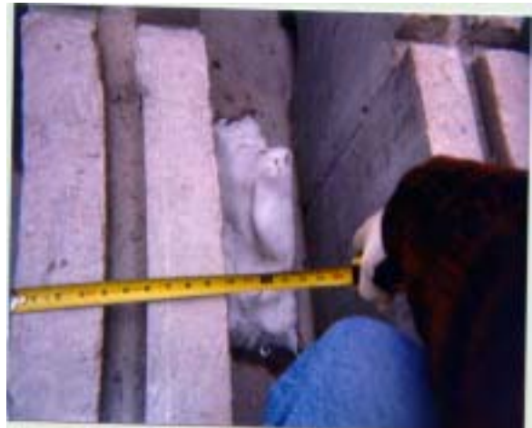
10" Support Beam w/2" Drain Channel
