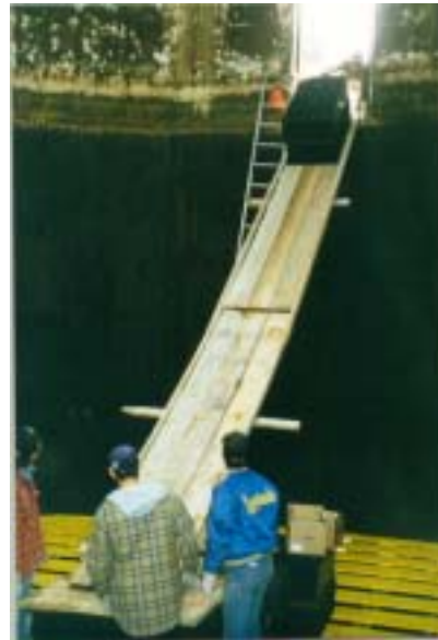
Wooden slide to tank floor for installation
