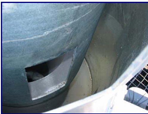
Figure 6 Discharging weir on the stationery supporting pier
