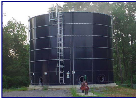
Figure 8 Ventilation openings on the base of the filter
