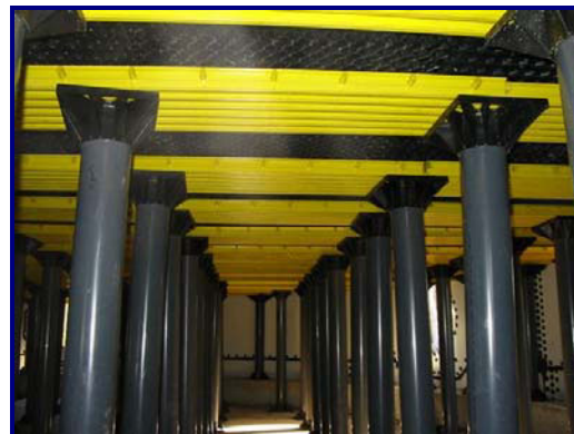
Figure 10 Column and pier media supporting system
