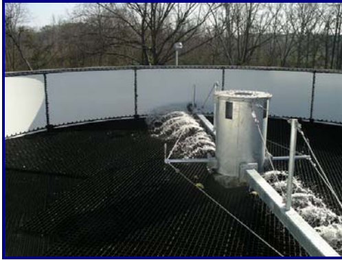
Figure 4 Overview on the hydraulically propelled distributor
