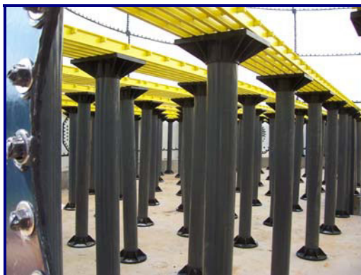
Figure 10 Column and pier media supporting system
